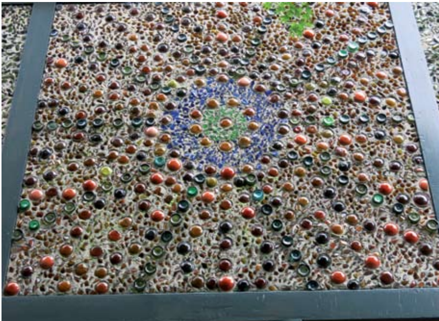
Embedded Glass on the Tilton House, McKim, Mead & White (1880-82).
