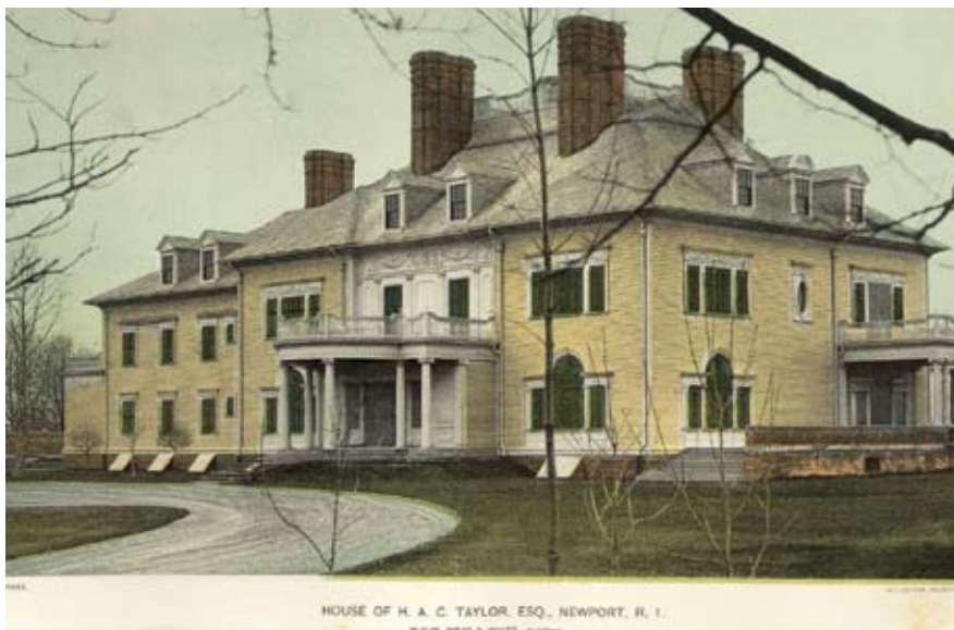
H.A.C. Taylor House; McKim, Mead & White (1882-84), Newport.
