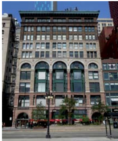
Fine Arts Building, Solon Beman, 1885-87 and 1897-98, east elevation. Photo by John H. Waters
