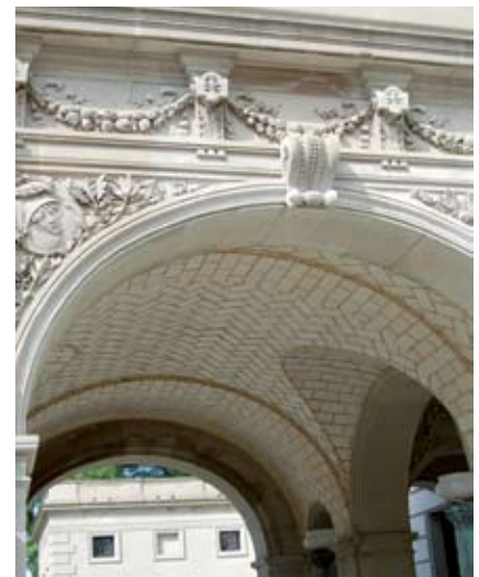
The Breakers, loggia with Guastavino vaulting; Richard Morris Hunt, 1882-95. Photo by Richard Guy Wilson
