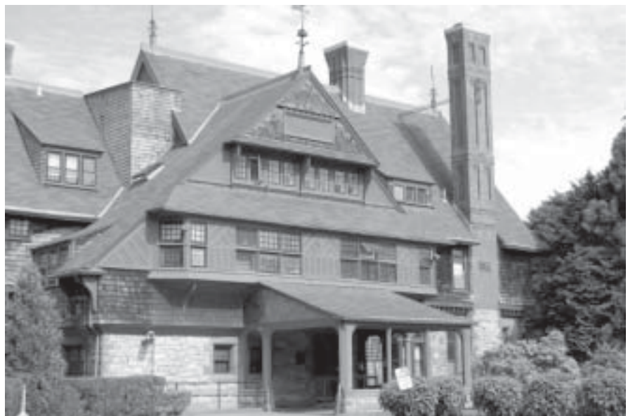
William Watts Sherman house, Newport, Rhode Island. (Henry Hobson Richardson with Stanford White, 1874-76, remodeling, McKim, Mead & White, 1880-81, c. 1900 addition by Dudley Newton). Photo: Richard Guy Wilson.
